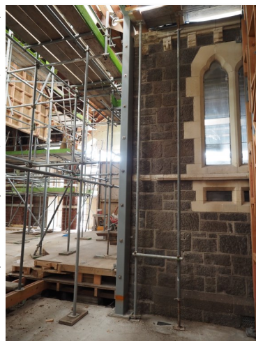
Reinforced south wall of the old sanctuary at the organ pit
