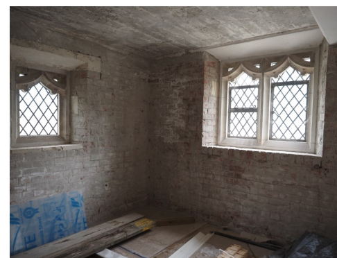
Inside the choir vestry the cracked plaster finish is gone from the walls, and cracks in the brick walls has been repaired
