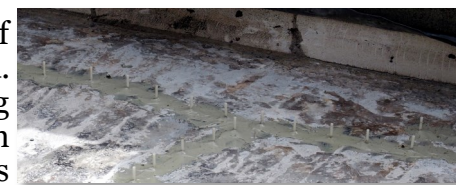
A section of repaired cracking in the bell-tower roof
