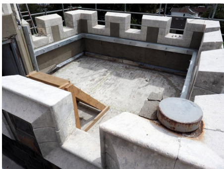
Top of the bell-tower wall secured with a band of steel pinned into the stone.
