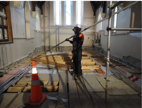
View into the chapel as a worker dismantles internal scaffolding. Note that the chapel floor is being rebuilt at a level below the original. On the floor behind him is a new window frame to be fitted into the north transept roof.
