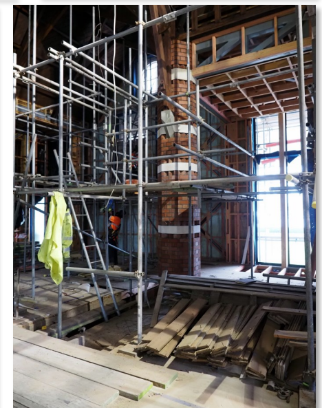
View of the new pillar in the south transept. Note the steel beam for roof support and one of the new windows streaming light into the choir space.
