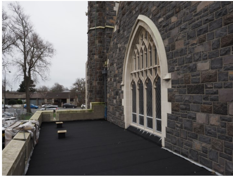
The completed roof above the new parenting room and toilets (with the two ventilation outlets).
