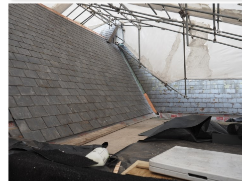
Looking under the white cover over the south transept, the roof has been substantially finished. The slates are new tiles from Wales, UK.
