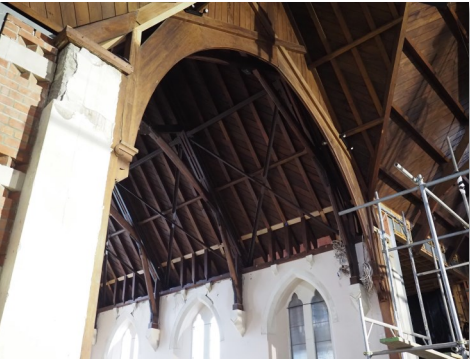
The chapel roof has been strengthened with the addition of a set of steel frames between the existing wooden rafters.
