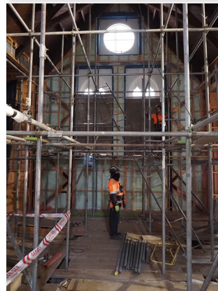
View of the south transept wall with the new window frames. The round frame is for the amazing blue Bill Sutton rose window.
