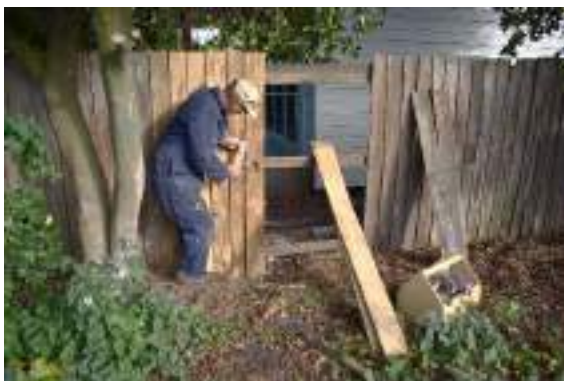
Anthony repairing an internal fence
