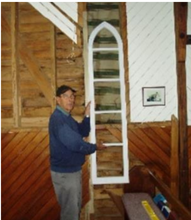
Brian Anthony replacing a rotten window frame at St Luke's
